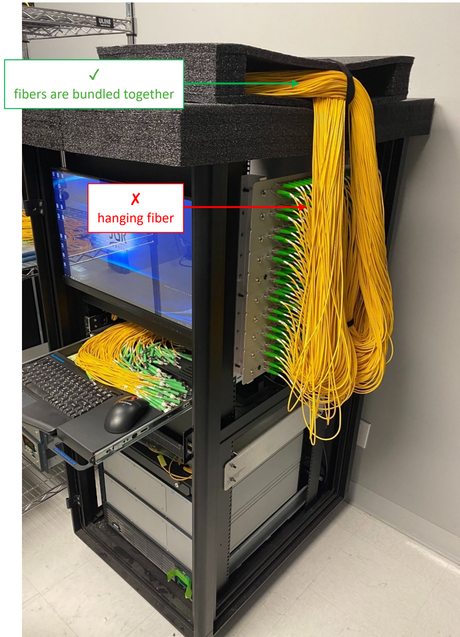
Figure 4: Fiber management example #2
